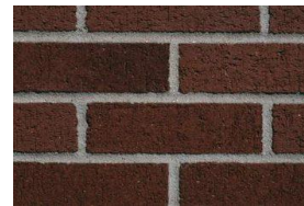
Raked joints have a uniform depth
